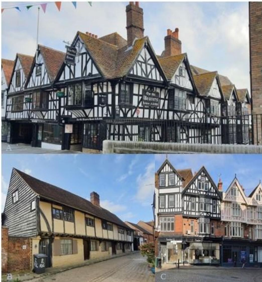
Figure 1.4 Examples of Wealden Style Terraced Houses. A. The Three Storey Old Weavers House dating to the 14 th century (name given based on Flemish and Huguenot weavers who settled in Canterbury during the 16 th and 17 th centuries). B. Example of Three Storey Terraced Houses on All Saint's Lane near High Street. C. Example of Four Storey Terraced Houses Across from the Entrance of the Cathedral.
